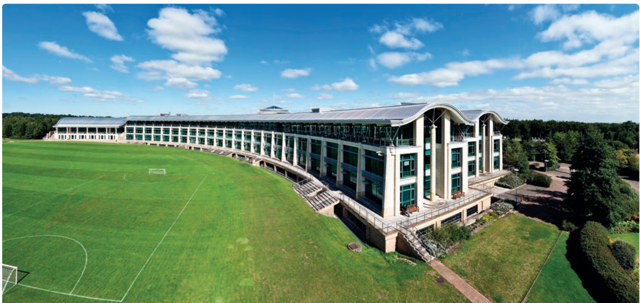
New roof at Wythall office allows for greater flexibility, power generation and operational efficiency
